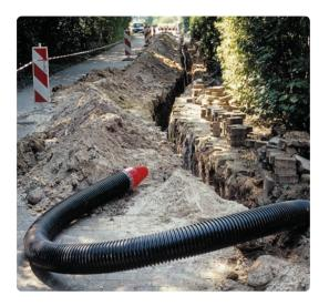
compacted layer for layer, from 500 mm the coverage must also be compacted by machine. Then place the routing barrier tape and fill in the trench. The jacket pipes remain stable under earth and SLW (heavy traffic load) of h=0.5 m up to max. 6 m. The required static evidence is verified according to the current regulation ATV-DVWK-A127 for embedded pipes. The verification applies only to certain installation conditions.
