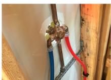
PEX is more forgiving and it's lighter than copper. We used to use CPVC, stainless and copper pipes, but ProPEX fittings, man, it's quick and fast.
