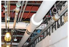
The ProPEX fitting is nice because it doesn't restrict the flow like insert fittings do.
