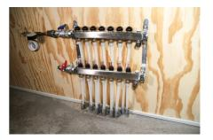
Besides offering a higher flow velocity compared to CPVC or copper, a PEX system holds a smaller volume of water than the same-sized system using either of these materials in the same pipe diameters.
