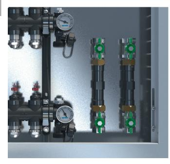
The factory has an appropriate fitting made of plastic with KTW certification. If no water meters are used, the fitting can be replaced with a fitting made of suitable metallic materials.
