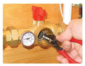
Step 3: Remove the circlip which retains the filter.
