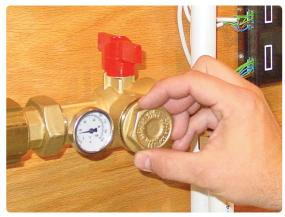
Step 5: Remove any dirt and debris from the filter.
