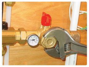
Step 2: Remove the filter-inspection cap.
