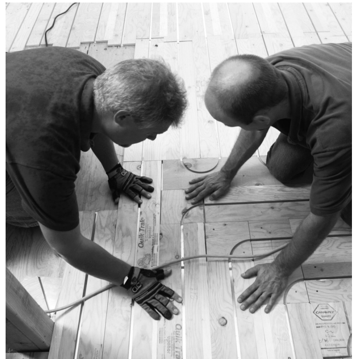
Figure 4: Installing Quik Trak straight panels
