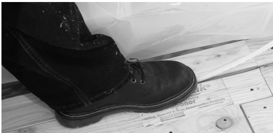
Figure 29: Use hard-soled boots or shoes to walk the tubing into the panel groove.
