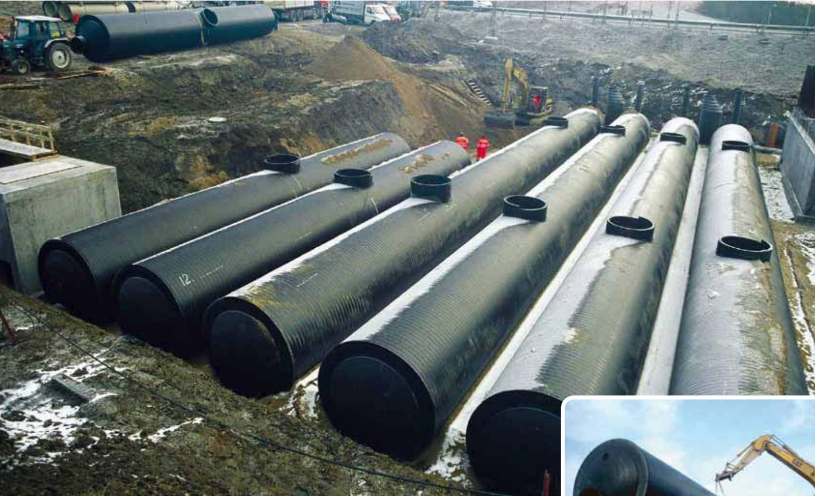
6 x 36 m of DN/ID 2,400 mm Weholite pipe, capacity 977 m<sup>3</sup>
