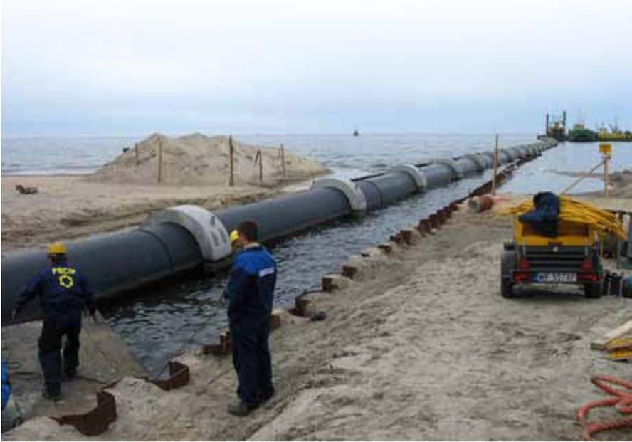
Tugboats transported the whole pipeline to its destination, where it was sunk in a carefully selected place.
