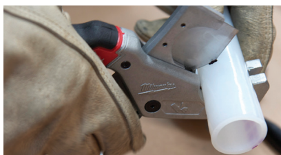
Figure 3-28: Cut Pipe at Marking
