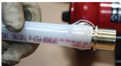
Figure 3-24 : Chauffer le raccordement
