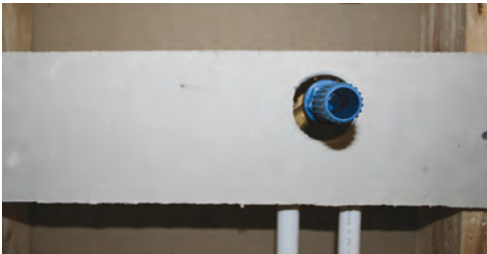
3 – Finish the wall over the assembly
