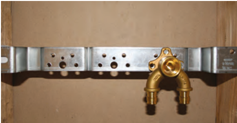
1 – Fix bracket and mount fitting
