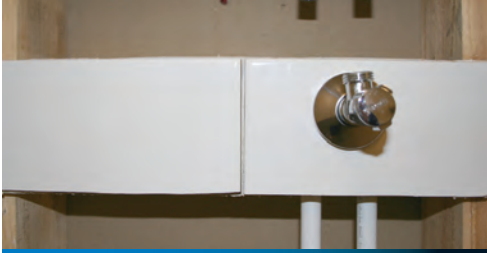
4 – Connect tap to the BSP thread.
