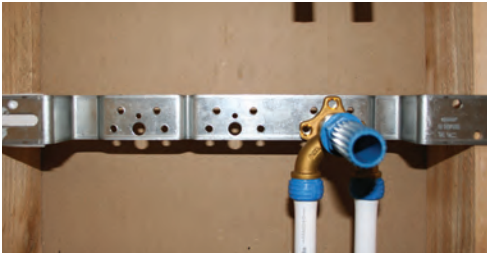
2 – Connect pipe and pressure test
