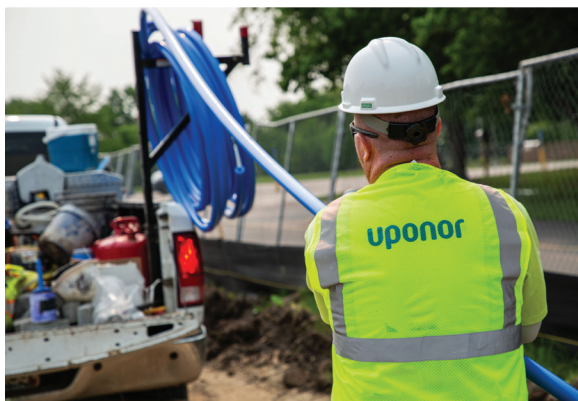
Figure 1 : Installation de tuyaux ServicePEX
