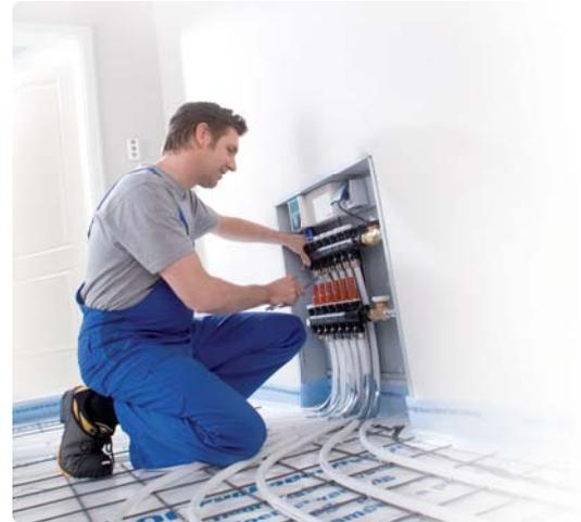
Thanks to this modular concept, the Uponor PRO 1" allows for easy manual push-in connection of manifold bases and tool-free reconfiguration for various connection options.
