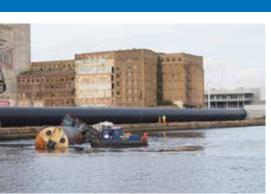
Weholite is a fantastic solution that can be used in a number of different applications. A welded system in diameters up to 3500mm, with associated tanks, chambers etc. Always with the possibility of adapting the customer's needs. Weholite is highly suitable for marine installations, since the unique pipe wall construction can be filled with ballast material.
