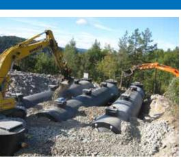
WehoPuts wastewater treatment plants for 10-60 households are delivered from the factory ready to install; the only thing that needs to be done at the site is to connect electricity and sewage.
