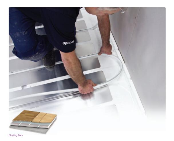
This is a system developed for larger areas and giving a soft floating floor. 30 or 50 mm thick for Uponor pePEX Q&E 20x2.0 mm.
