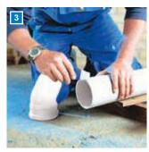
After that, the permitted insertion depth, minus the expected thermal expansion is marked on the end of the pipe, and a lubricant, designed for plastic waste water pipes with connectors and rubber seals made from EPDM, is applied to the end of the pipe.
