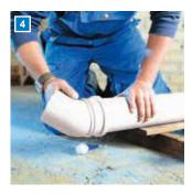
The pipe is then inserted into the sleeve, up to the insertion mark. The thermal expansion of the pipe must be taken into consideration when making all the junctions and connections.
