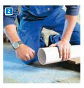
Then the end of the pipe is deburred on the inside and the outside. The ends of the pipes must not have any longitudinal scoring. The sealing groove and the sealing ring of the sleeve must be clean and free of any damage.
