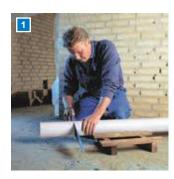
The pipe is cut at right angles with a fine-toothed (1-2 mm) saw or cutting device which is specially designed to cut plastic waste water pipes.
