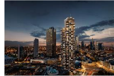
Decentralised heating and cooling for the tallest residential building in Germany Grand Tower, Frankfurt, Germany
