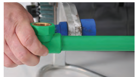
Figure 2-5: Allowing the fused joint to cool undisturbed
