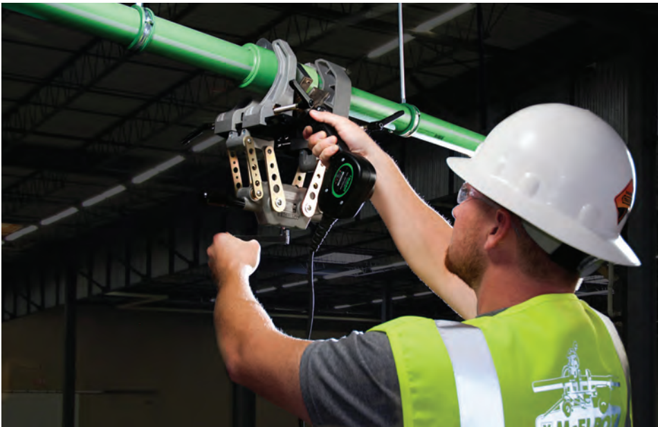
Figure 5-1: Making overhead PP-RCT connections
