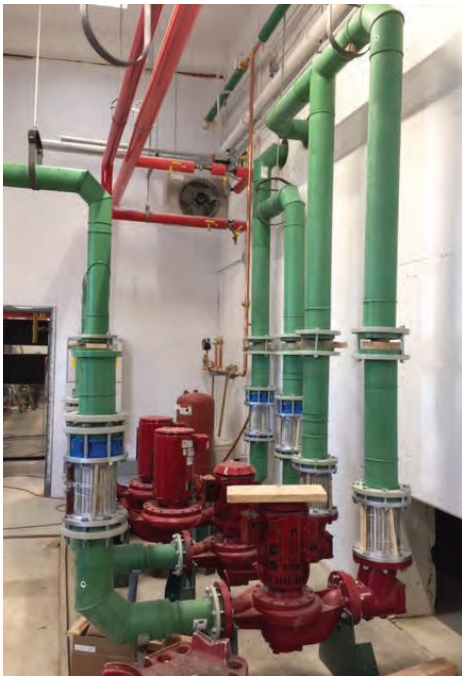
Figure 1-5: PP-RCT mechanical-room piping
