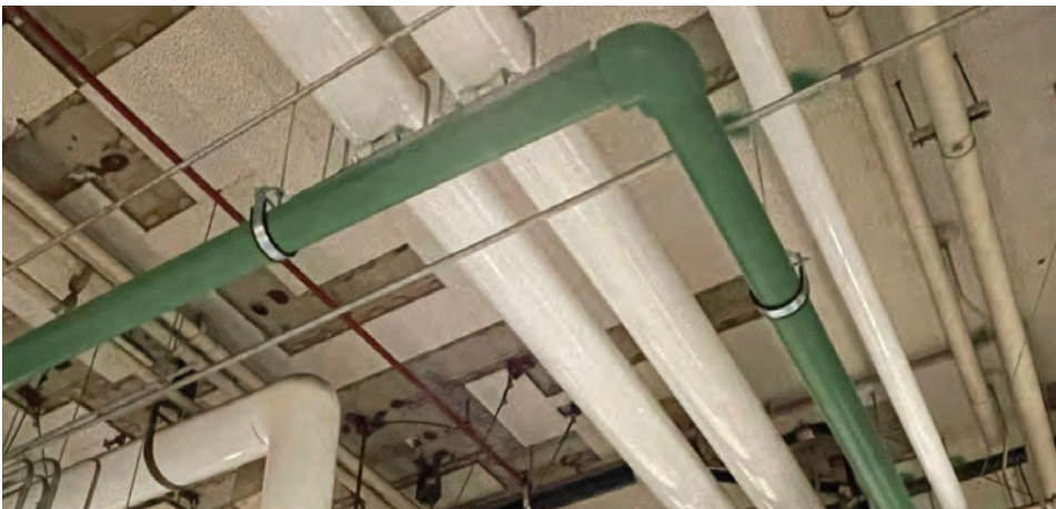
Figure 5-2: Supporting Uponor PP-RCT piping
