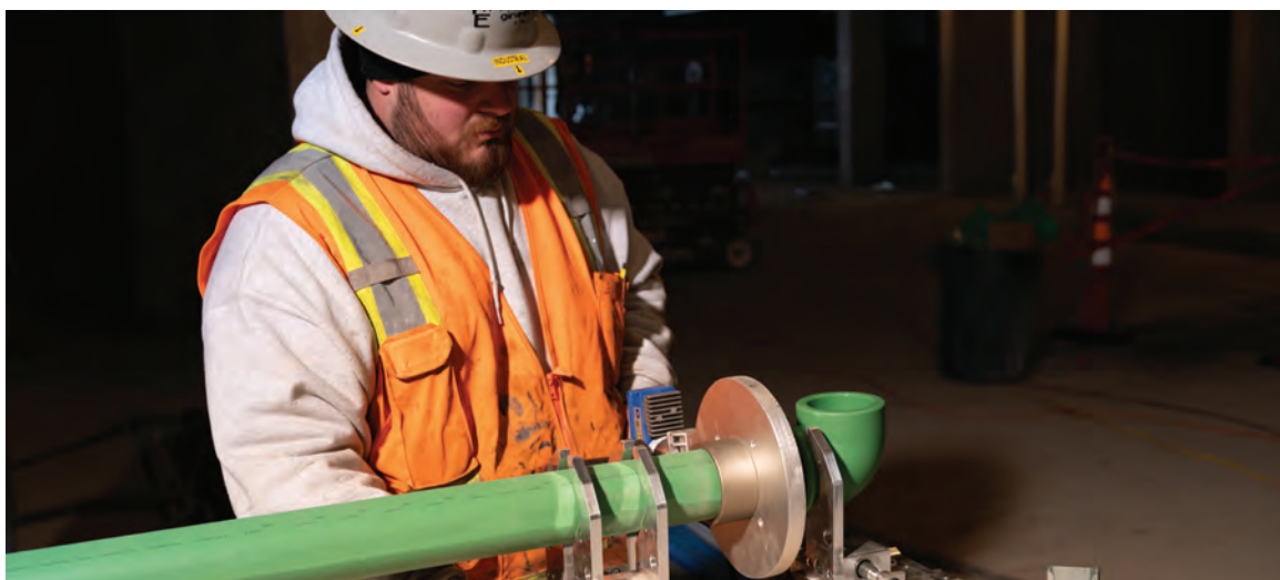
Figure 2-1: Heat-fusion connection
