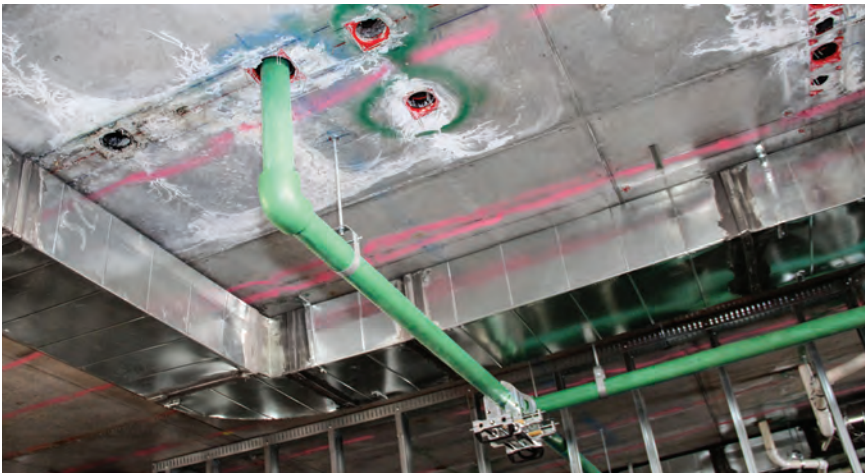
Figure 3-1: Ceiling penetration
