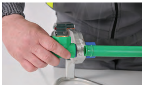
Figure 2-4: Connecting the pipe and fitting
