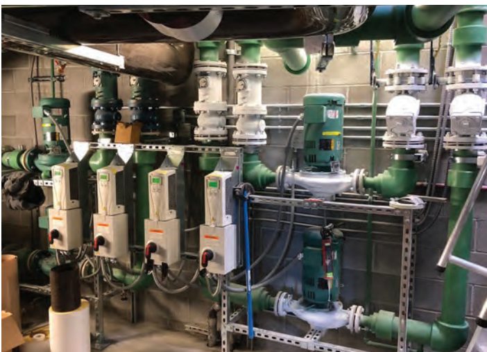
Figure 1-3: PP-RCT mechanical-room piping
