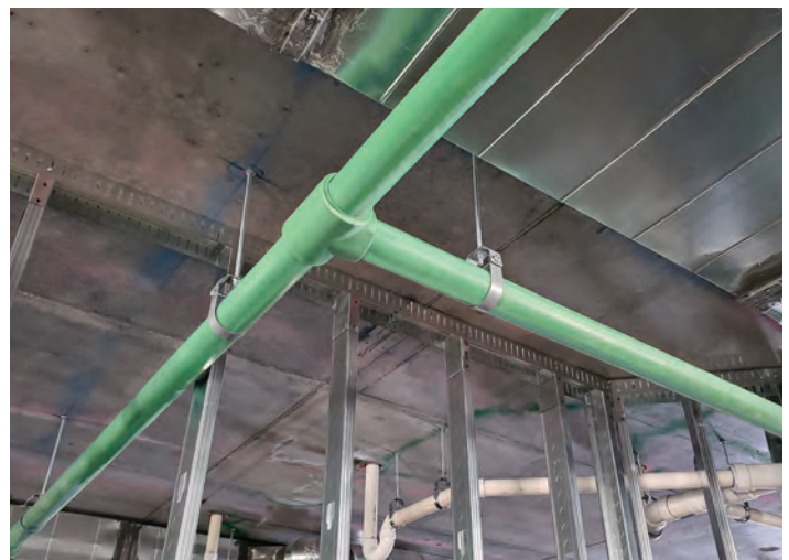
Figure 1-4: PP-RCT suspended piping
