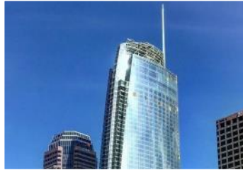
Radiant cooling system for the world's largest concrete pour in the 10 th tallest building in the USA: Wilshire Grand, Los Angeles, USA
