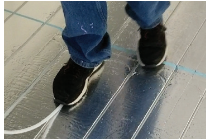
Figure 13: Press pipe into the groove
