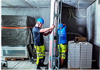
Prefabricated Uponor Riser Port for quick and easy installation – and quick repair, if necessary - in a 6 floor apartment building: Helsinki, Finland
