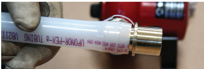
Figure 2-35 : Chauffer le raccordement
