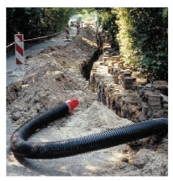
conditions, are suitable for loading by heavy traffic (SWL 60 = 60 t) according to worksheet ATV-A 127. The ring stiffness of the jacked pipe ist proved according EN ISO 9969 to be able to withstand 4 kN/m<sup>2</sup> (class SN4).
