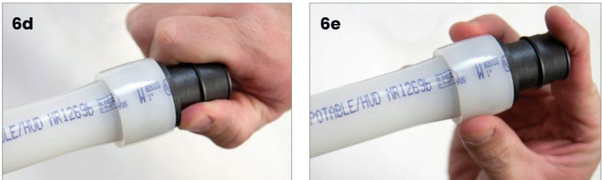
**Figure 4-7:** Inserting ProPEX fitting into 1" Uponor PEX piping
