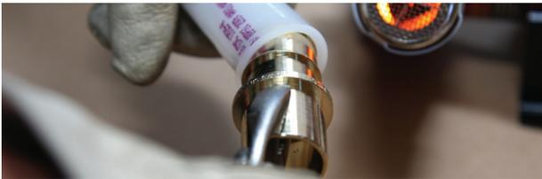
**Figure 4-27: Work piping back and forth**
