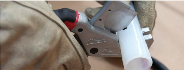
**Figure 4-30: Cut pipe at marking**
