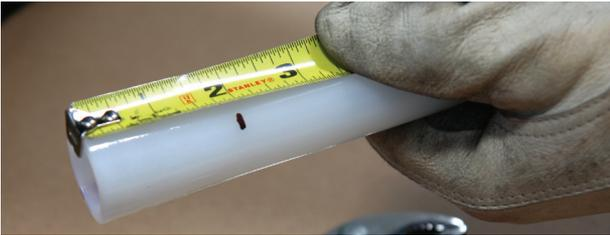
**Figure 4-29: Measure from end of pipe**
