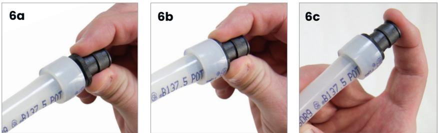
**Figure 4-6:** Inserting ProPEX fitting into 1/2" Uponor PEX piping
