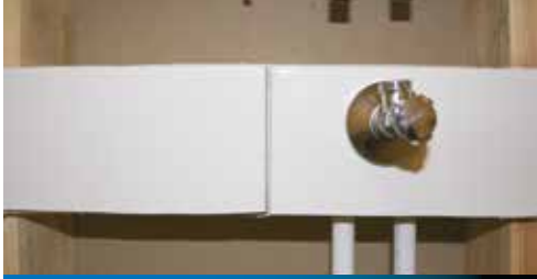
4 – Connect tap to the BSP thread.
