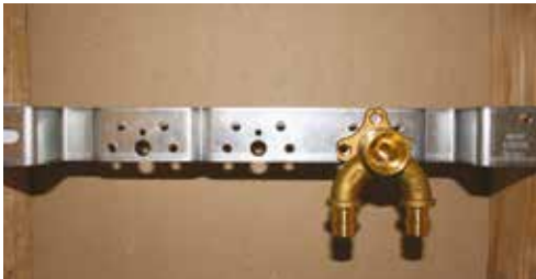
1 – Fix bracket and mount fitting
