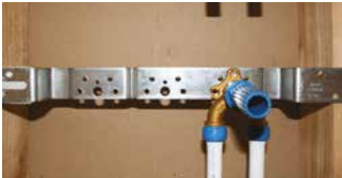
2 – Connect pipe and pressure test
