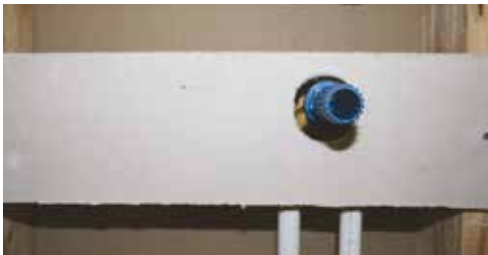
3 – Finish the wall over the assembly
