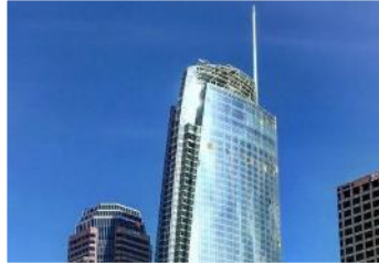
Radiant cooling system for the world's largest concrete pour in the 10 th tallest building in the USA: Wilshire Grand, Los Angeles, USA
