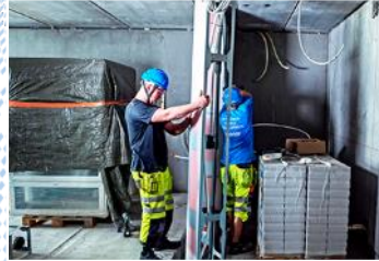
Prefabricated Uponor Riser Port for quick and easy installation in a 6 floor apartment building: Helsinki, Finland
