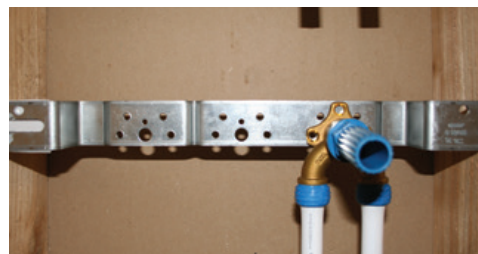
2 – Connect pipe and pressure test
