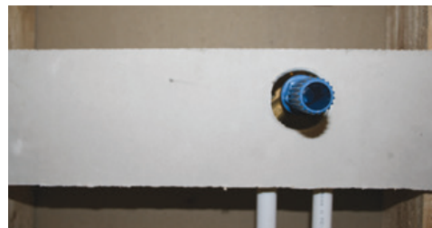
3 – Finish the wall over the assembly
