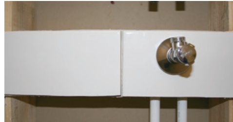
4 – Connect tap to the BSP thread.
