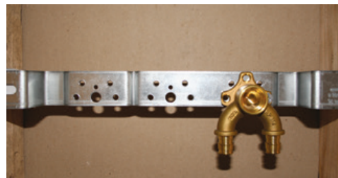
1 – Fix bracket and mount fitting
