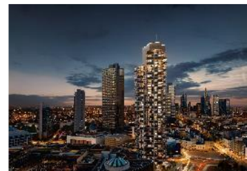
Decentralised heating and cooling for the tallest residential building in Germany Grand Tower, Frankfurt, Germany
