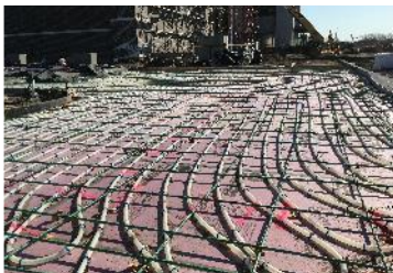
Scheels department store saves energy costs with radiant heating and improves safety with snow/ice melting Minnesota, USA
