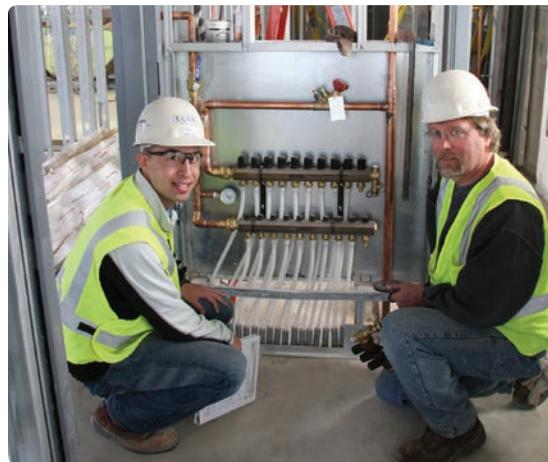
Figure 4-3: Manifold in Flush-mounted Wall Cabinet
