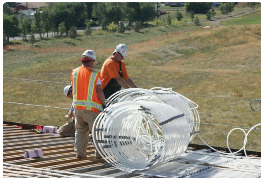
"Zones on this project ranged anywhere from 48 to 250 feet long and up to 24 feet wide," Barela explains. "We customized each mat in whatever dimensions were needed." For example, on the widest zone, four 6-foot mats were connected to complete that zone.
