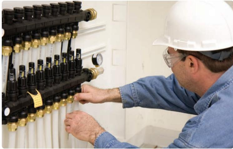
Figure 4-13: Uponor Engineered Polymer (EP) Manifold
