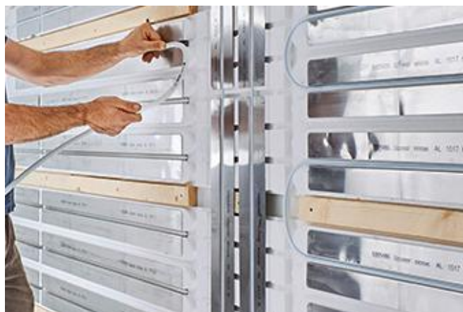
Uponor Siccus heat conducting lamellas – stable aluminium lamellas with omega groove for optimal heat transfer to the system pipe 2-fold pre-punching for simple shortening without tools of the lamella size 120 x 1180 mm.
