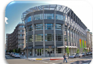
The David Brower Center, Berkeley, California (Leed Platinum) - Uponor's in-slab hydronic H/C
