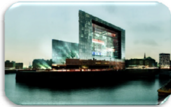
Headquarters of the Spiegel Media Group, Hamburg - Uponor radiant Heating/Cooling with Thermally-Active Building Structures (TABS)
