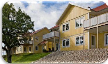
High-quality/low-budget housing in Stenungsund, Sweden - 44 residences with Uponor heating and plumbing
