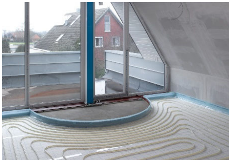
Radiant heating and cooling
