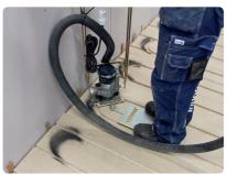
Use the Uponor milling machine to make grooves or use specially made truning plates.
