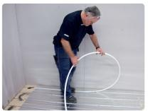
The pipes are positioned and fixed in place in the heat emission plates.
