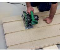
The panels are easily cut with a circular saw.
