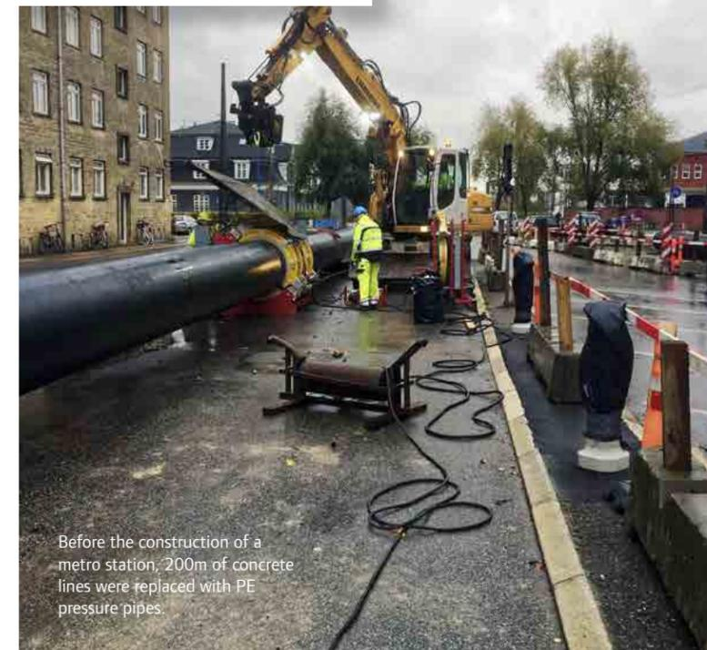
Before the construction of a metro station, 200m of concrete lines were replaced with PE pressure pipes.
