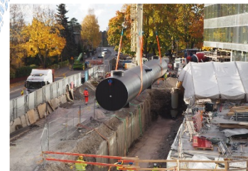
Weholite stormwater tank to attenuate runoffs at the new Children's Hospital: Helsinki, Finland
