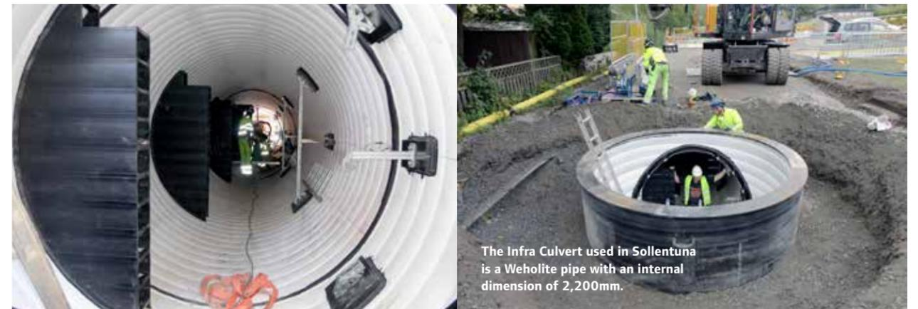
The Infra Culvert used in Sollentuna is a Weholite pipe with an internal dimension of 2,200mm.
