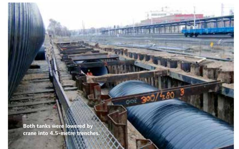
Both tanks were lowered by crane into 4.5-metre trenches.
