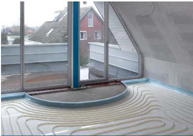
Radiant heating and cooling
