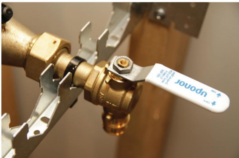
**Figure 19: Uponor ProPEX LF Brass Elbow Water Meter Valve**
