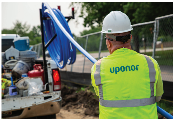
Figure 1: Uponor ServicePEX pipe installation
