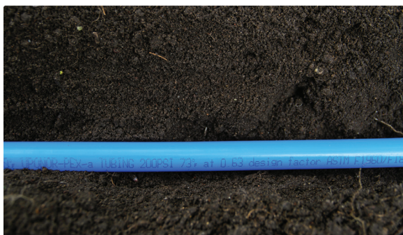
Figure 5: Uponor ServicePEX temperature and pressure rating on pipe
