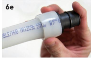
**Figure 27: Inserting ProPEX fitting into 1" Uponor PEX piping**
