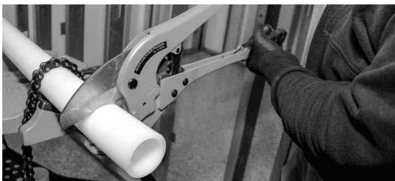
**Figure 14: Ratchet-style pipe cutter**
