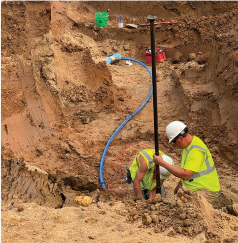
**Figure 11: Install Uponor ServicePEX in a snaking pattern with sufficient slack in the line to allow for contraction due to temperature change prior to backfilling.**
