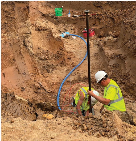
Figure 11: Install Uponor ServicePEX in a snaking pattern with sufficient slack in the line to allow for contraction due to temperature change prior to backfilling.
