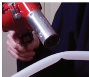
Figure 32: Reforming kinked piping
