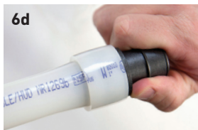
Figure 27: Inserting ProPEX fitting into 1" Uponor PEX piping
