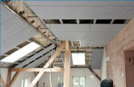
Wall and ceiling heating systems like Uponor Renovis can complement an underfloor heating system. Besides, they are especially interesting when modernizing attics.
