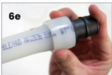
**Figure 6: Inserting ProPEX fitting into 1" Uponor PEX piping**
