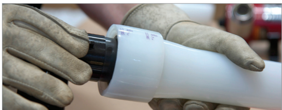
Figure 26: Insert fitting
