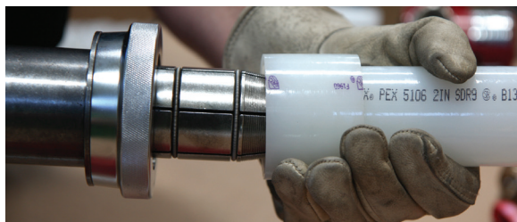
Figure 22: Slide head into piping
