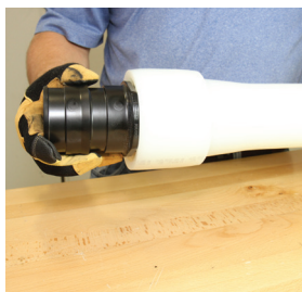
Figure 19: Insert fitting
