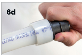
Figure 6: Inserting ProPEX fitting into 1" Uponor PEX piping
