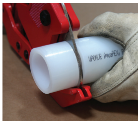
Figure 20: Cut pipe
