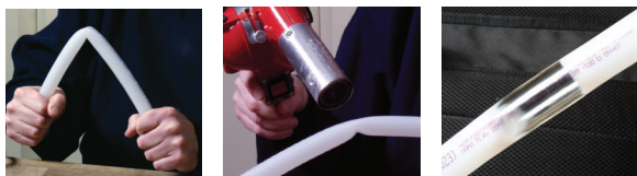
Figure 43: Reforming kinked piping
