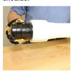
Figure 19: Insert fitting
