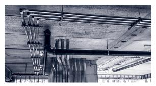
Figure 55: Supporting PEX with PEX-a Pipe Support
