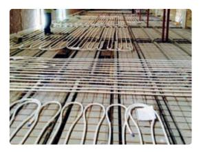
Uponor Contec system installation with ribbed slab
