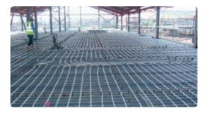
Uponor Contec installed in metal deck
