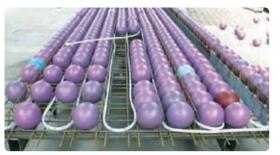
$\mathsf{Cobiax}^{\otimes}$  modules, coupled with Uponor Contec system as precast modules
