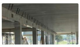
Uponor Contec modules incorporated into precast hollow core
