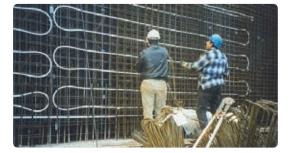
Uponor Contec modules installed in wall
