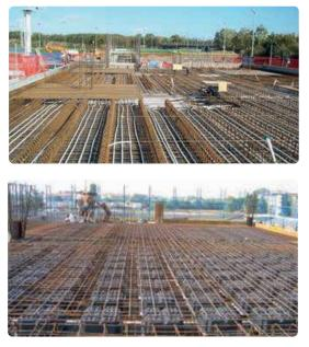
Uponor Contec installation, concreting and U-Boot modules installation
