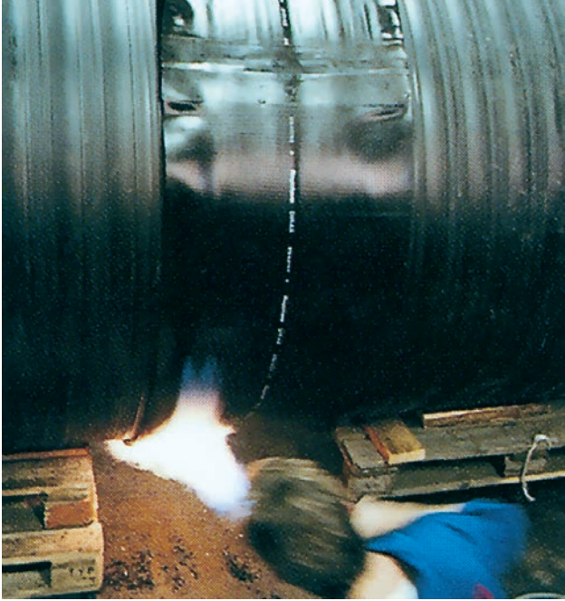
Heat shrink sleeve installation
