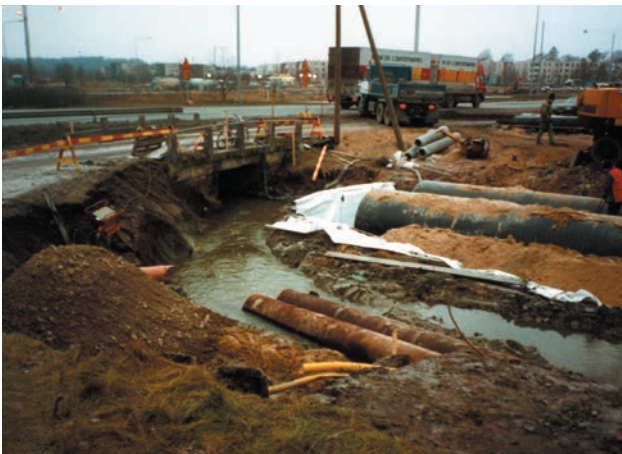
Helsinki, Finland: At the roundabout on the Ring 1 main road, the cover depth is only 400mm. Weholite SN4 DN/ID 1600mm, 2 parallel culverts.
