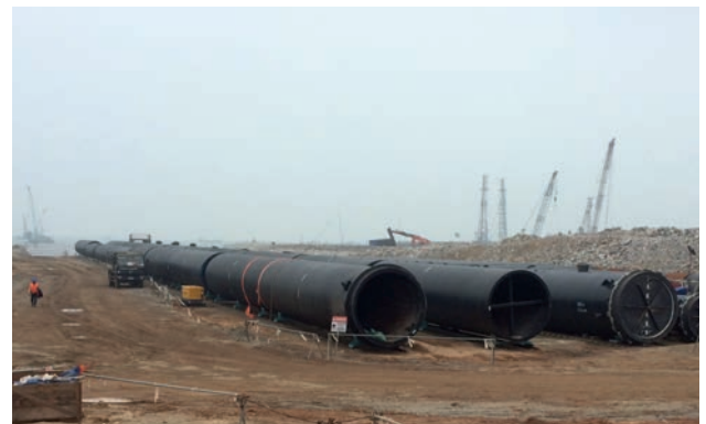
Nghi Son, Vietnam: Marine outfall for the oil refinery, Weholite DN/ID 2700mm and 2025mm. The total supply included engineering and design, welding and profile filling, together with installation supervision.
