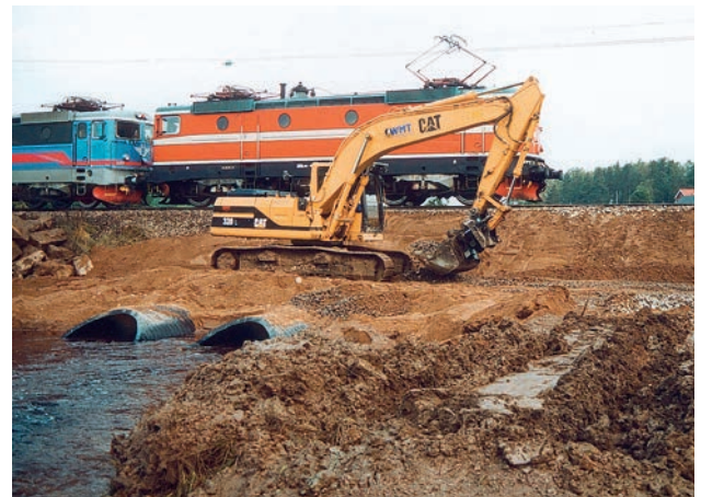
Degerfors, Sweden: Railway culverts Weholite DN/ID 1800mm, 2 × 24m.
