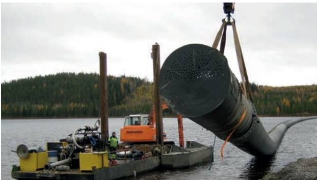
Talvivaara mine, Sotkamo, Finland: Uponor submerged a 250m long Weholite DN/ID 1600mm pipe as raw water intake pipe.
