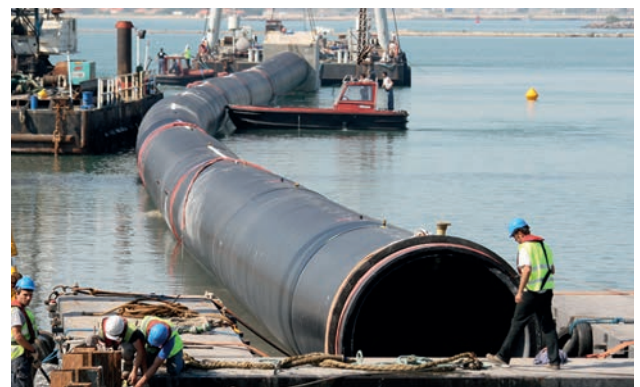
Fos-sur-Mer, France: Cooling water pipelines for a power plant were delivered as a turnkey project. Weholite pipes DN/ID 2200–2400mm were installed to a total length of 1260m. Installation length 206m, Ballasting inside the profile wall.
