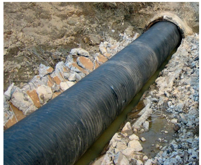
Hämeenlinna, Finland: A highway crossing was renovated by sliplining a Weholite pipe DN/ID 1000/1125mm into a concrete pipe DN 1300mm. Jointing type: Extrusion welding. Total length 750m.
