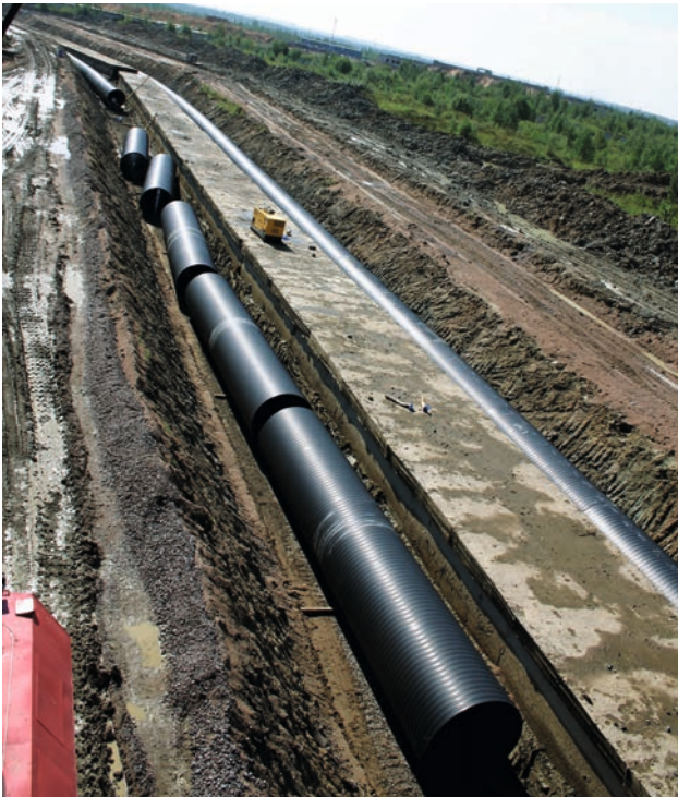
St. Petersburg, Russia: Weholite pipes DN/ID 2000mm were installed as outfall pipeline for a wastewater treatment plant. Of the 1400m length, 200m is marine pipeline. Weholite was also used in the starting end of the pipeline, at railway crossings and to extend old steel-, and concrete pipes. Additionally, several hundred metres of DN/ID 50 – 2000mm PE and Weholite pipes were delivered to the site.
