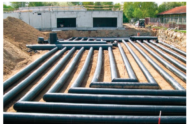
Sønderborg, Denmark: Collector pipes for geothermal air heating under a school building. Installation length 16m, installation depth 2m.
