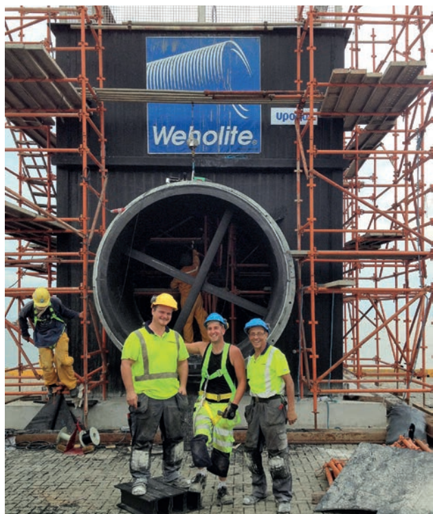
Philippines, intake tower
