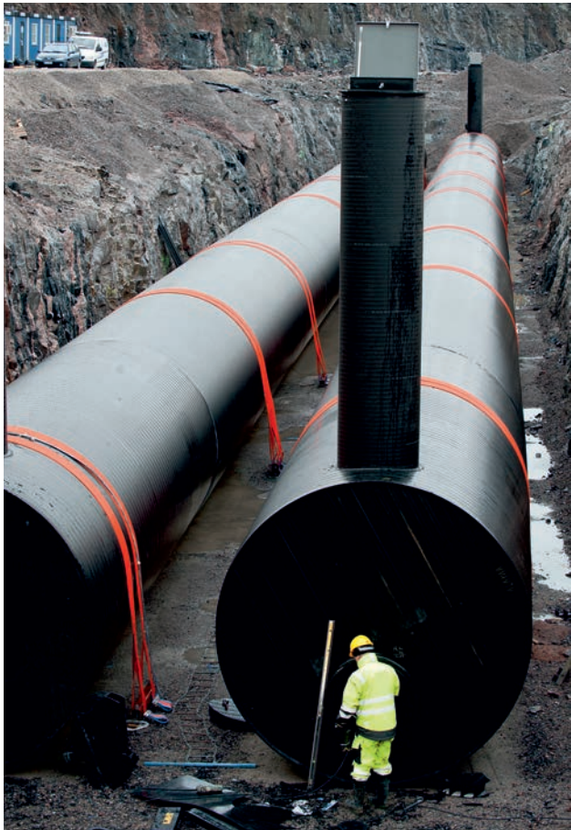
A stormwater retention tank for the energy company Vantaa Energy in Finland. The tanks were made of Weholite pipes DN/ID 3000mm in lengths of 20m. These 20-metre pipes were welded on-site to two tanks of 100 metre each.
