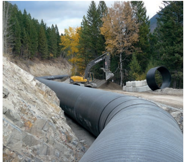
Aberfeldie, B.C., Canada: During the renovation project for the Aberfeldie Run-of-River hydroelectric power plant, 855m DN/ID 3000mm Weholite pipe, PN 1.5 bar was installed as well as 14 bends and 2 manholes DN/ID 1200mm.
