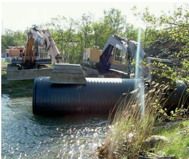
Åvabro, Åland Islands: An old corrugated steel road culvert was renovated by sliplining a Weholite pipe DN/ID 1600mm SN4, total length 30m.
