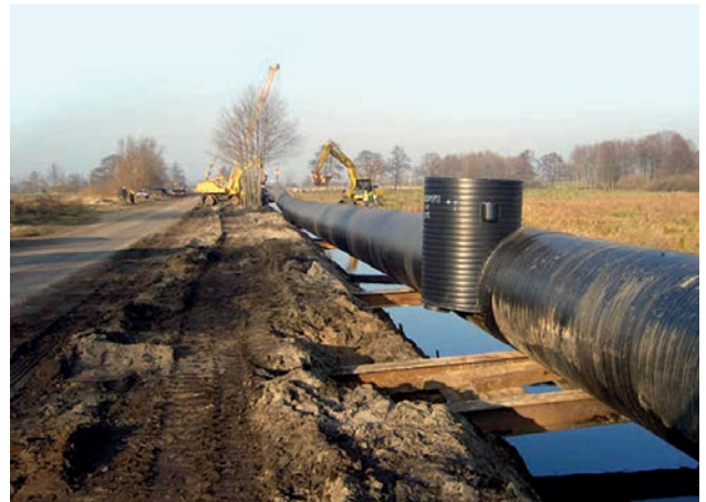
Gdynia, Poland: Wastewater treatment plant discharge pipes. Uponor delivered 2257m Weholite pipes DN/ID 1400–1500mm and 22 manholes. To facilitate installation, most pipes were delivered in 15m lengths.
