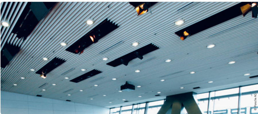
VARICOOL Opti Y as a flat high-performance lamellae ceiling
