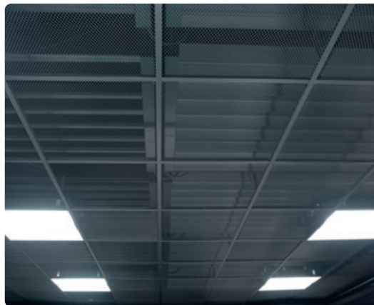
VARICOOL Opti Y as a cooling module above air permeable ceiling panels
