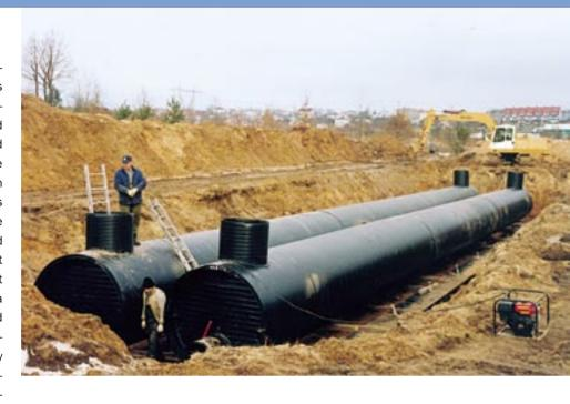
PE allow production of any manhole and fitting to order; very odd models tailor-made to optimize the properties and designs are often impossible to obtain in concrete.
