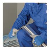
Divide the heat conduction plate simply by bending it
