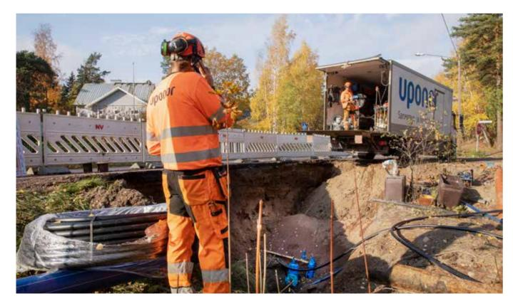
horizontal drilling and long lining, that is, methods in which pipe is installed underground or inside an old pipe. In such cases, there's always the risk that a depression or the like in the ground will subject the pipe to unusually high stress," says Kimmo Sjöman, Sales Manager at Uponor.
