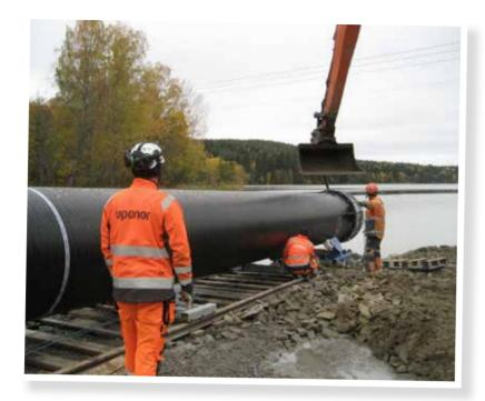
The district cooling plant under construction in Kuopio in Central Finland will be one of Finland's largest plants that utilises lake water. We holite Marine pipes – designed for underwater installation - ensure that the new plant's intake pipe, measuring almost two kilometres in length, and outfall pipe, itself slightly less than one kilometre long, will be installed rapidly, easily and safely in Lake Kallavesi.
