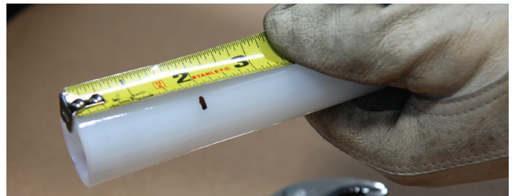
Figure 2-38: Measure from end of pipe
