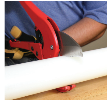
Figure 2-14: Cut pipe
