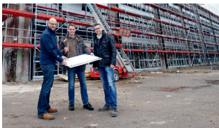
Uponor provided accurate planning in close co-operation with the general contractor
