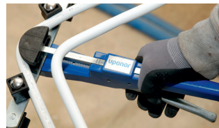
The MLC pipe Uponor Uni Pipe PLUS was used for the risers, loop installation and connection to the radiators
