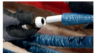
Special RTM fittings with integrated pressing function reduced installation time
