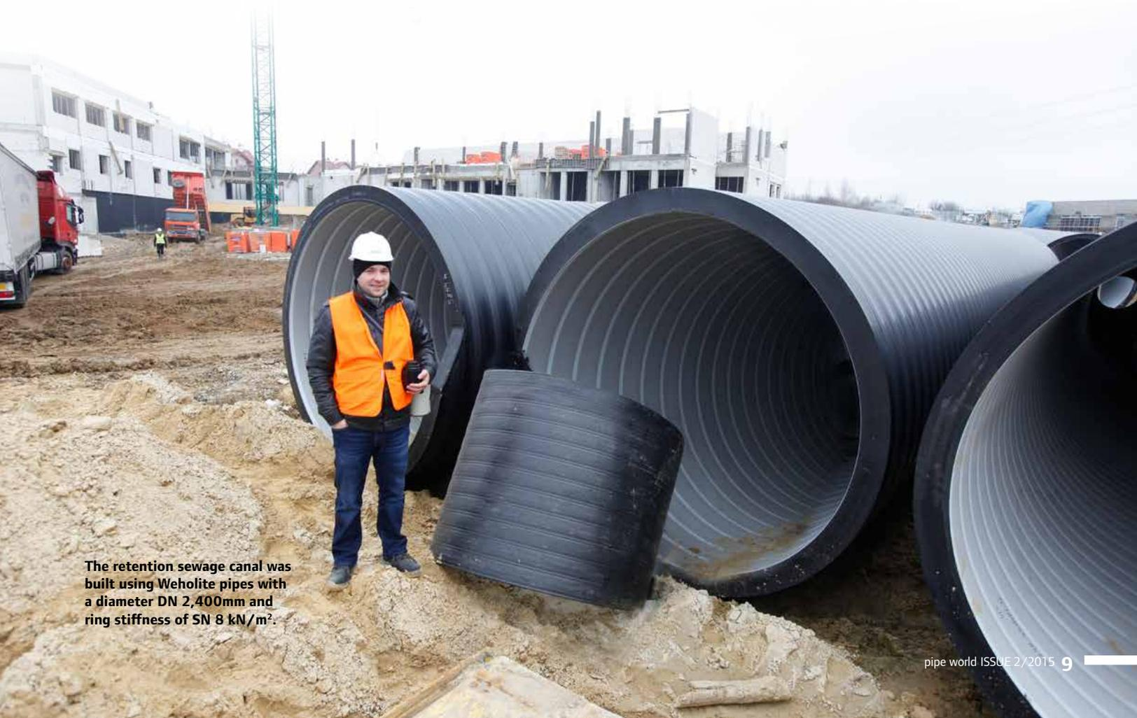
The retention sewage canal was built using Weholite pipes with a diameter DN 2,400mm and ring stiffness of SN 8 kN/m<sup>2</sup>.
